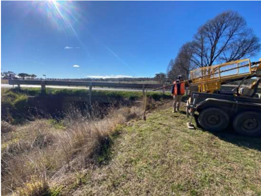
Location of BH04 - Facing northeast.
