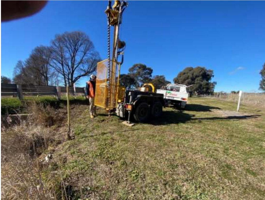
Figure 6: Location of BH04 adjacent to Muttama Creek in Gundagai Road easement immediately south of Nashs Lane intersection - Facing Southeast
