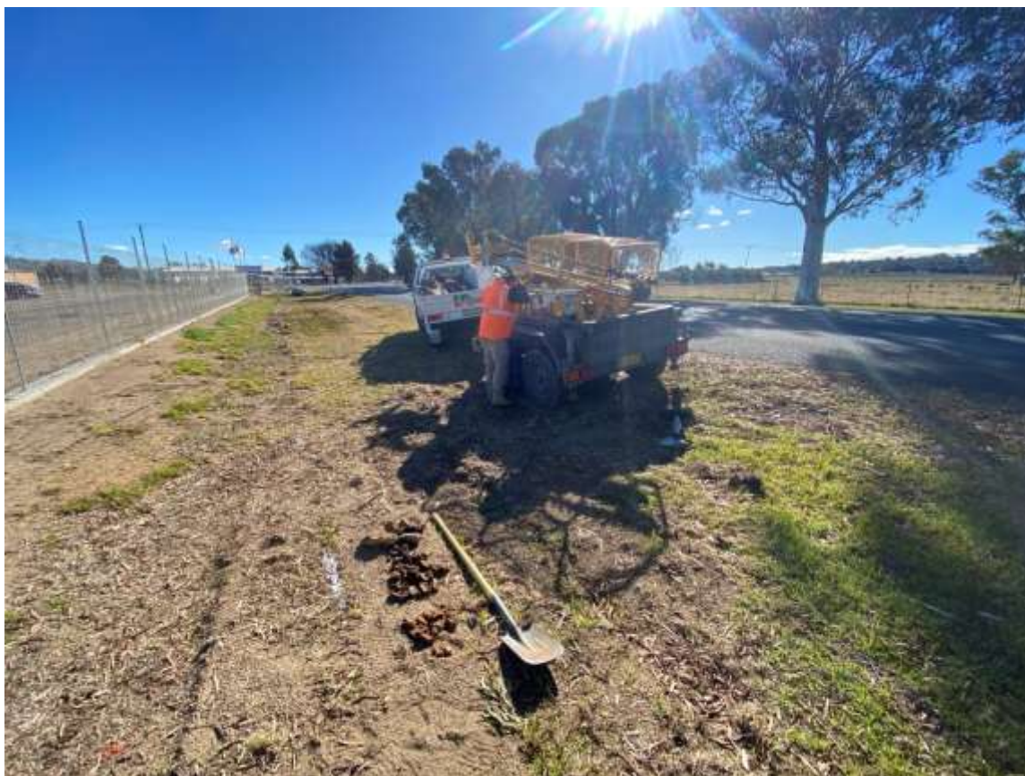
Figure 4: Location of BH03 in road easement in front of 107 Gundagai Road - Facing north.
