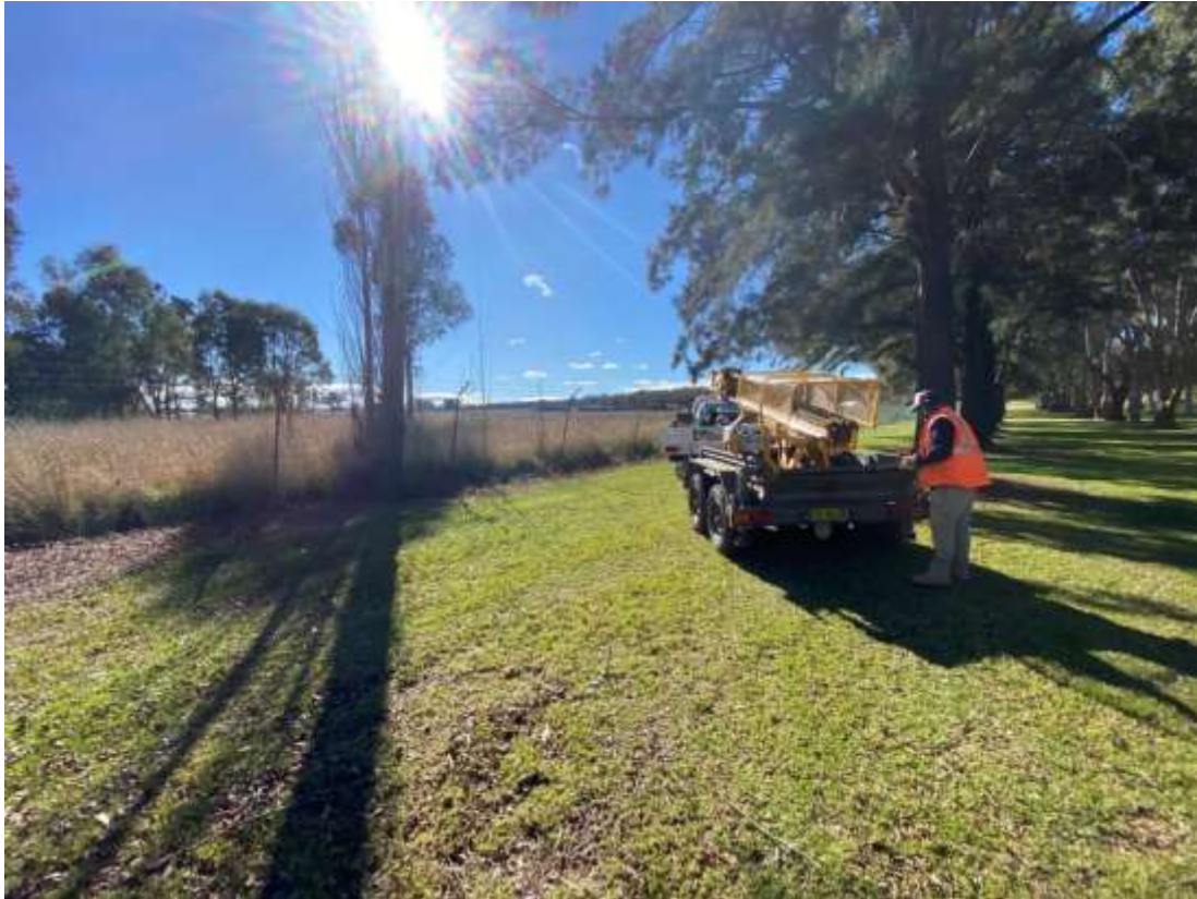
Figure 9: Location of BH05 in northwest corner of WWTP property adjacent to the Gundagai Road easement - Facing north northeast.
