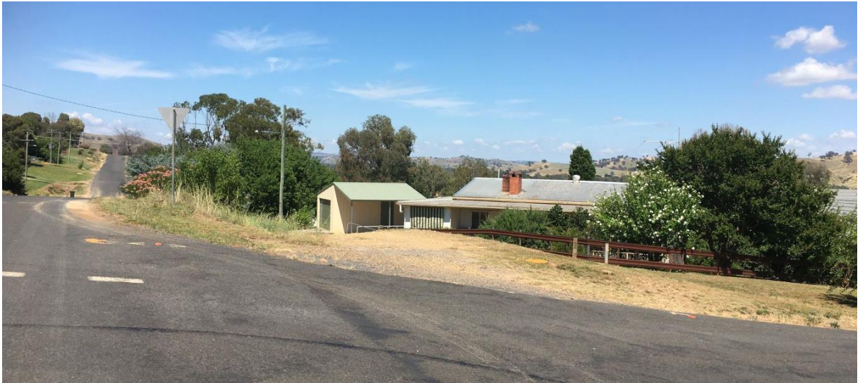
Figure 8 – Runoff into private property. Corner Luke St and Eagle St, South Gundagai (G7)
