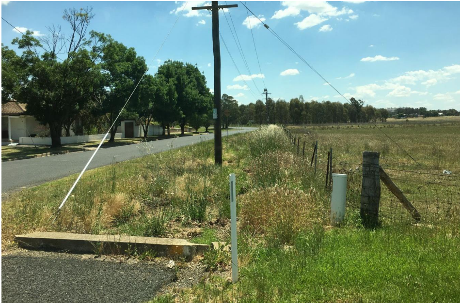
Figure 4 – Open roadside drains – Adams Street north of McGowan Street, Cootamundra (C5)
