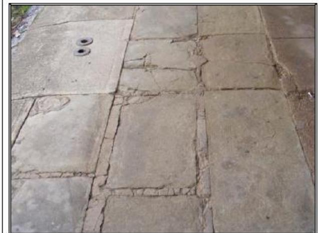
Condition 7 Extensive cracking and movement
